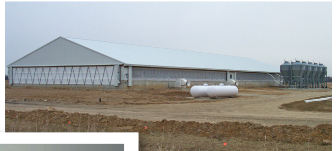
Wean to Finish Research Facility
